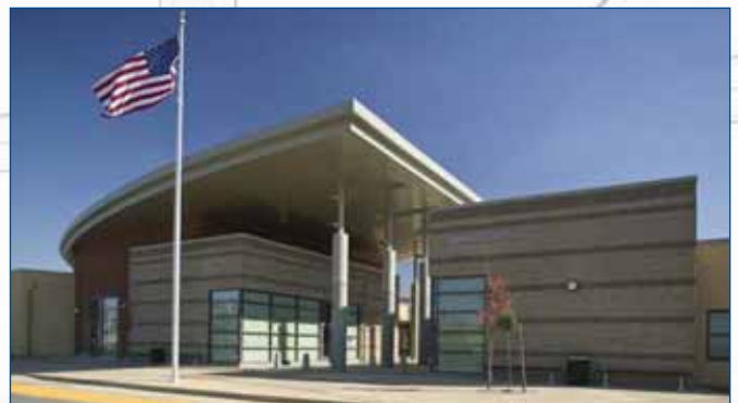
Vista del Lago High School Administration Building
