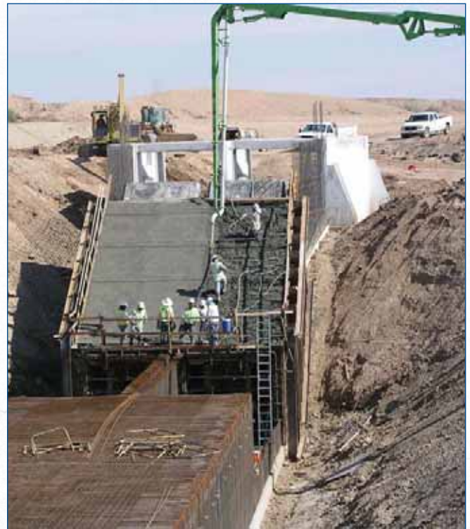
Construction of the Coachella Canal Lining Project
