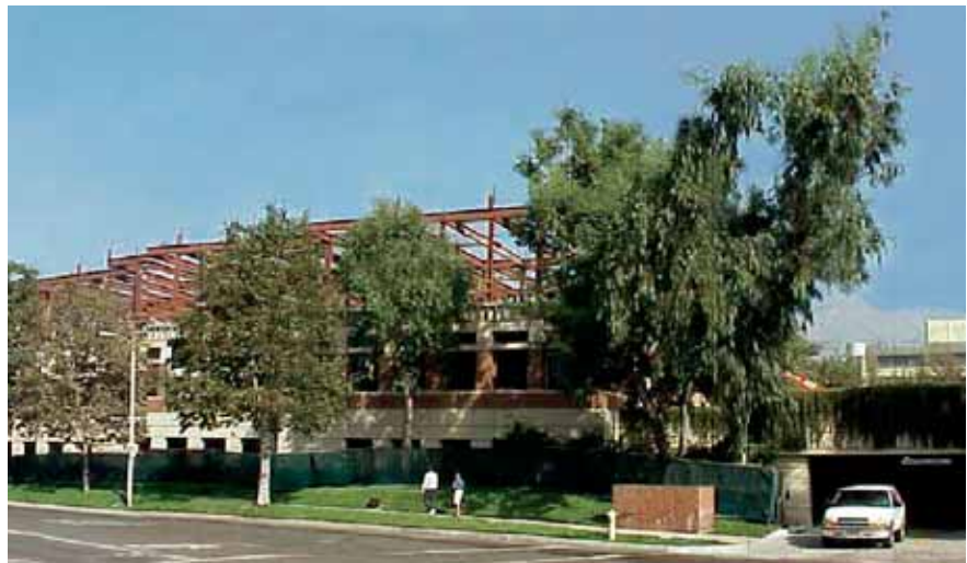
View During Construction
