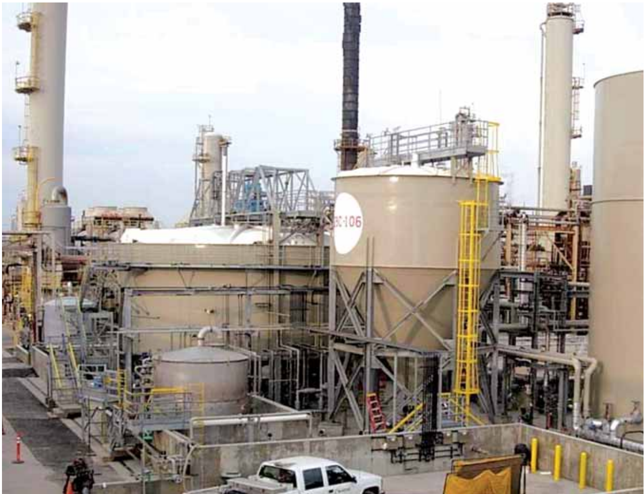
Torrance, Refinery Selenium Reduction Project
