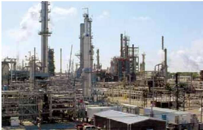
Marathon Robinson Refinery GDU Project
